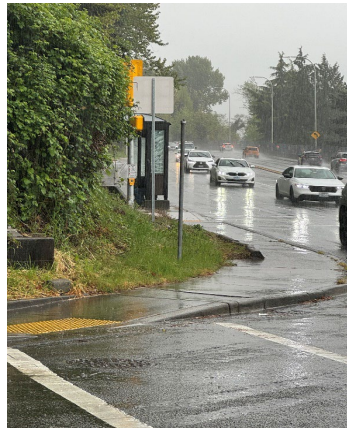
Existing Conditions along NE Sunset Blvd at Edmonds Ave NE (western project terminus)
