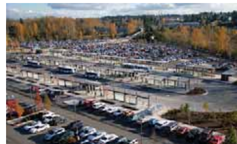
More than $800 million invested in transit centers, HOV direct access ramps and park-and-ride lots
